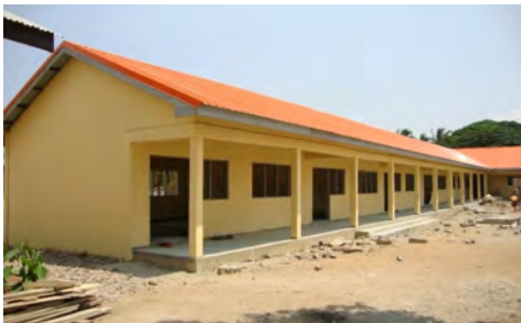
New Six Room Teaching Block
